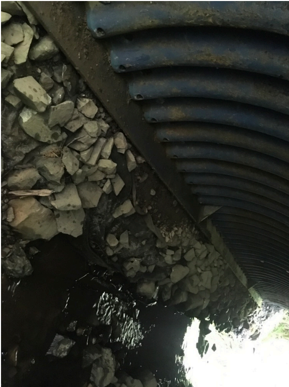
Left Bank Abutment when facing downstream
